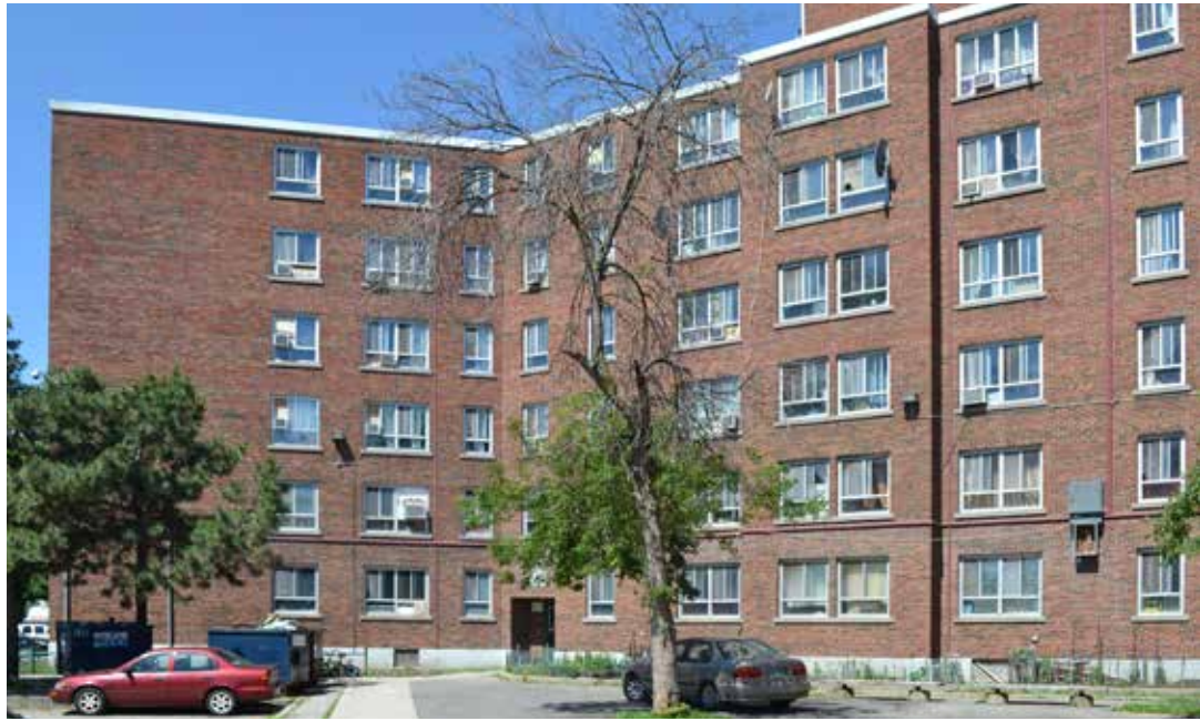
Regent Park 1940s building slated for demolition
