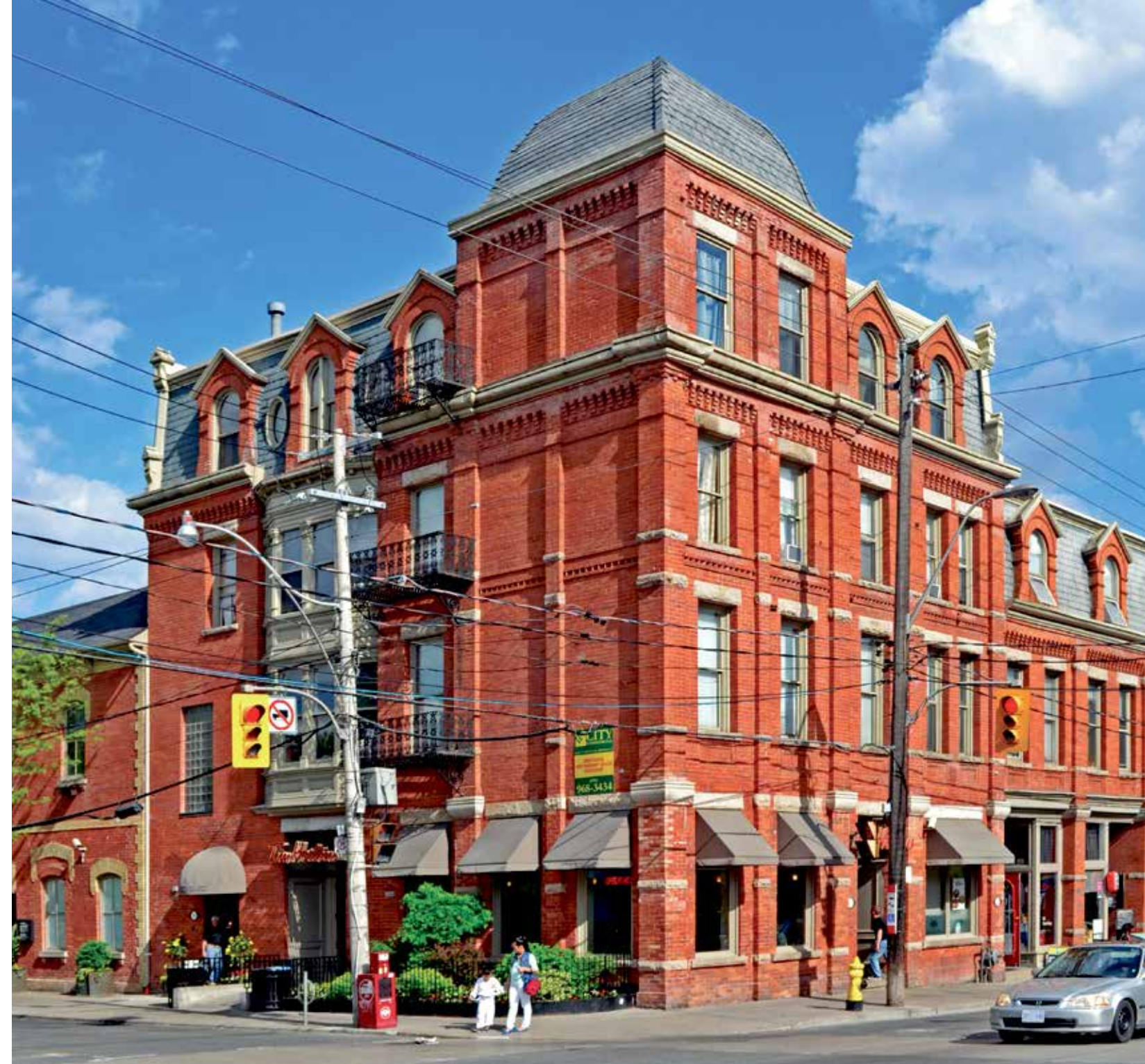
No longer a hotel, the Winchester Hotel (built in 1888) is one of Cabbagetown's most recognized landmarks.
